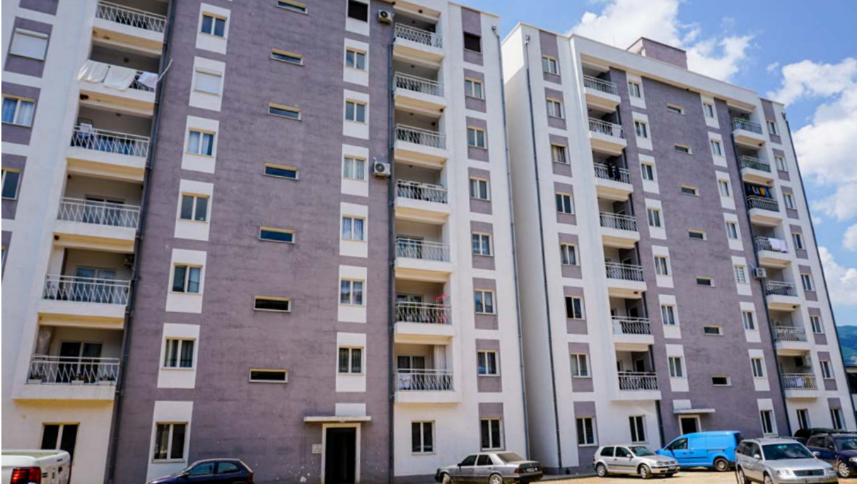
Picture 2 NHA low-cost housing complex in Kukës
